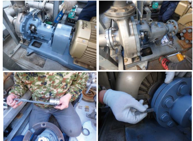
Fig. 1. Photograph of the RIBF Cooling water pump maintenance.
